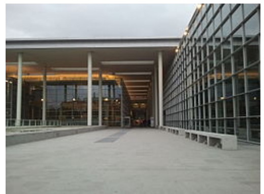
Careggi hospital in Florence.
